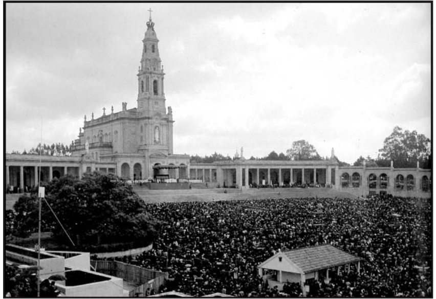
The small building in lower right hand corner, the little chapel (the Capelinha) is built on the exact spot of the apparitions.
